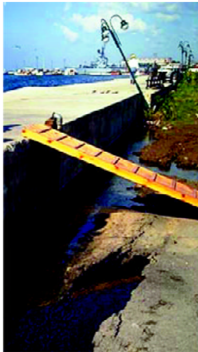
Settlement caused by liquefaction at the Izmit Public Marina. Taken from Earthquake Spectra, 1999 Kocaeli, Turkey Earthquake Reconnaissance Report
