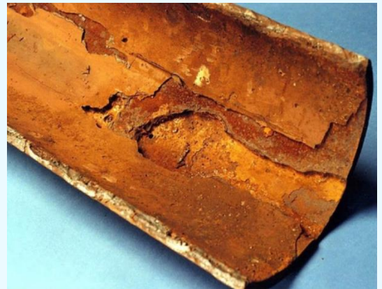
Internal corrosion in a crude oil pipeline
